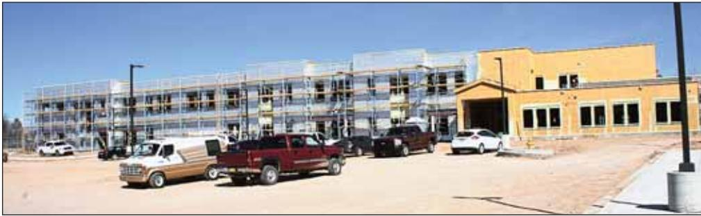
The outside work on the charter school building is progressing. Rigid insulation has been installed on the north end and the stucco base layer has been installed on the eastern and southern side of the buildings. Some of the islands and lighting have been installed in the parking lot.
